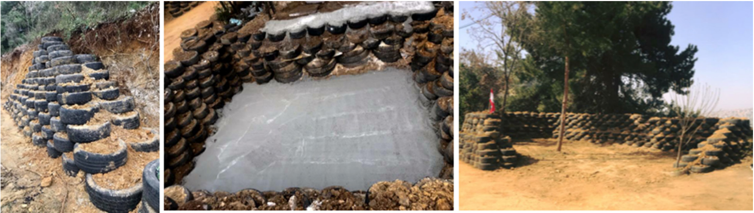
Figure 4. Construction of Wall with Unused Tyres. Source: BiClean Facebook Page.
